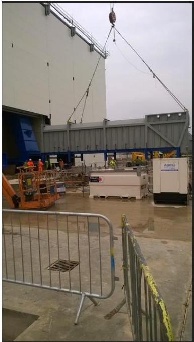
Installing the gasifier
